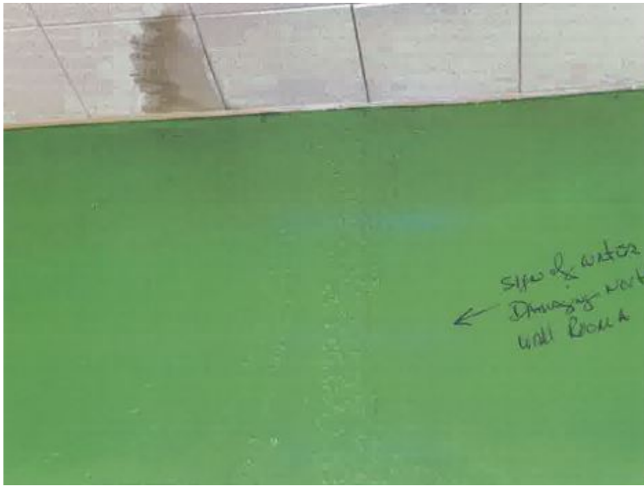
Room A – Ceiling and Wall
