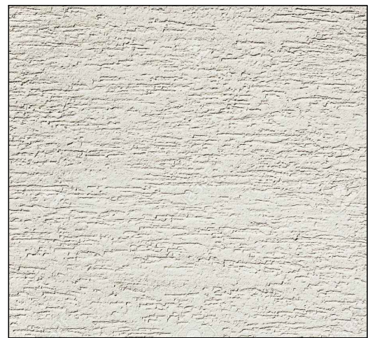
Keynote #2 STUCCO 2: 7/8" thick 3-coat Portland Cement Stucco: Smooth finish; finish coat to be hand applied. Color: Light gray.
