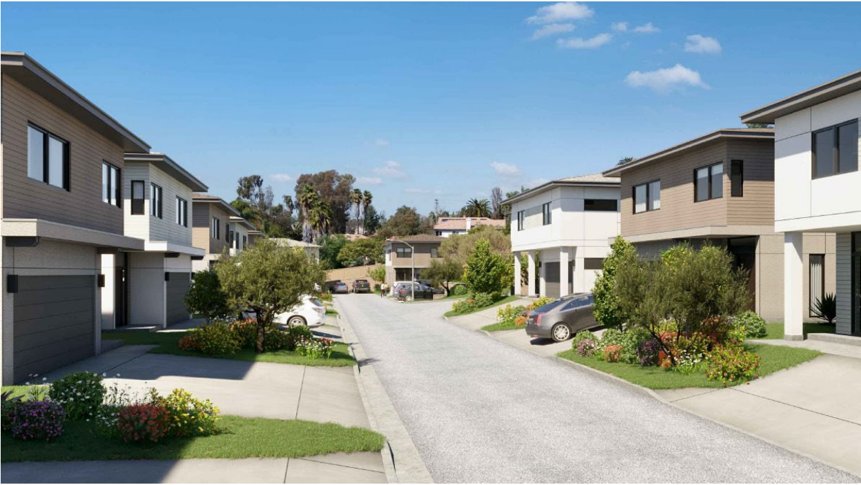
North facing elevation toward Sarajayne Lane
