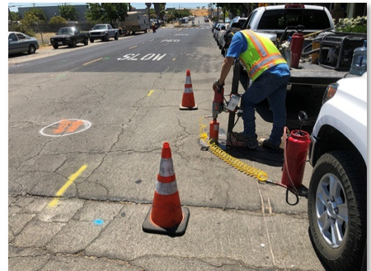
Field crews installing strategic traffic
