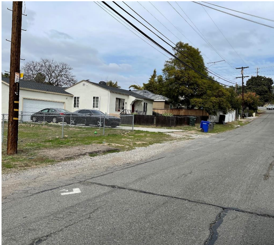
Example of deficiencies in the sidewalk network in residential areas of Lemon Grove. Lemon Grove residential areas could benefit from assessing access, safety, and connectivity.
